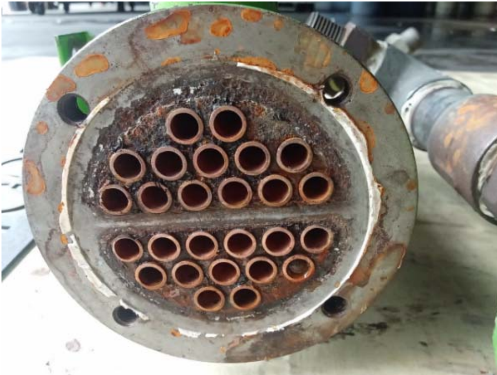
OIL COOLER BEFORE CLEANING
